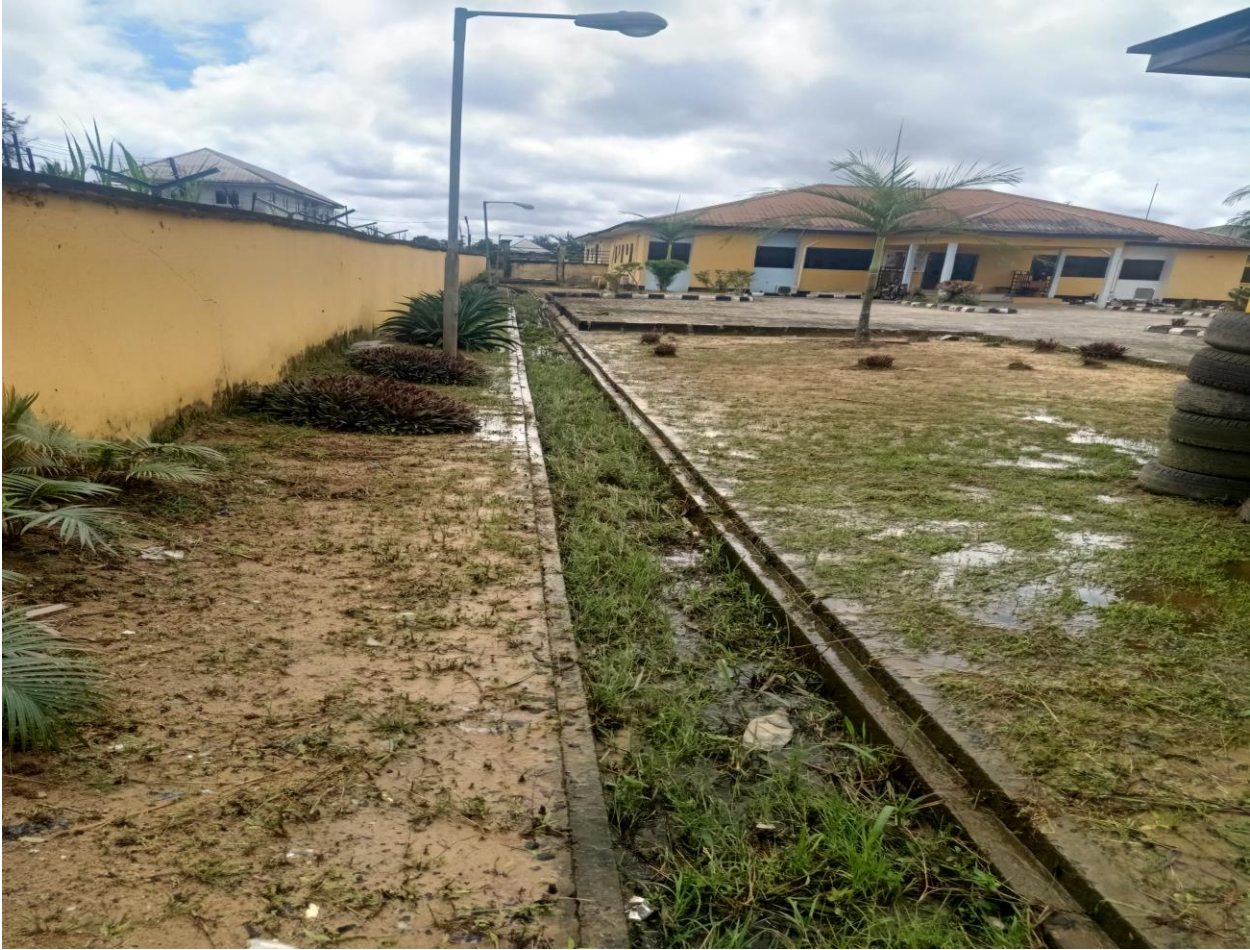
ZONAL INTERVENTION: Const of Waste water drainage @ Admin Block
